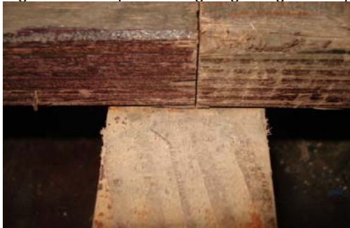
Fig 1: Correct positioning of gratings on support beams
