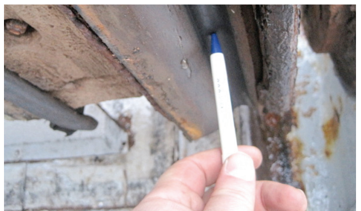
Ascertaining deformation on hatch sealing
